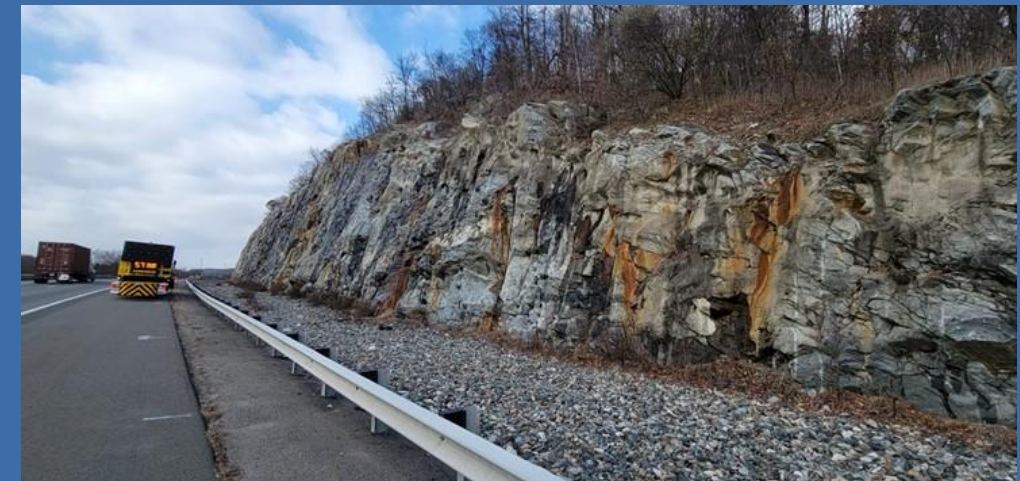
Example: Route 80 Westbound, Roxbury
