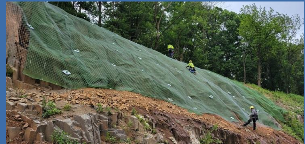
Example: Route 280 Westbound, West Orange
